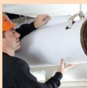
ASJ+ is moisture resistant to intermittent, short duration liquid water exposure such as precipitation during construction.\*
